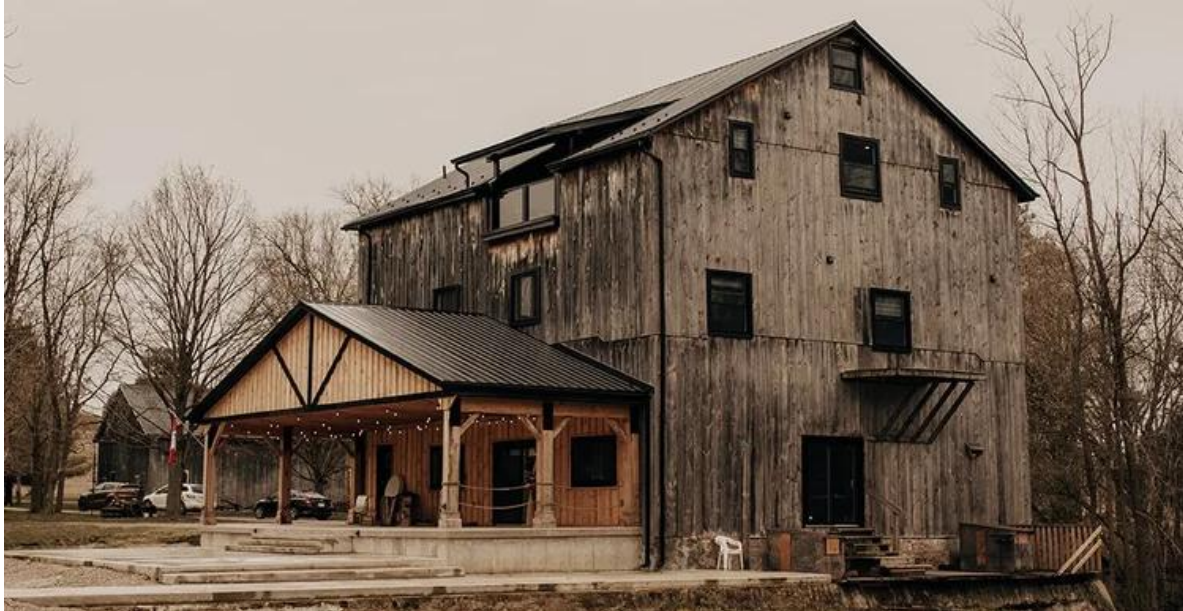
Figure 5-7. The Post and Beam Event Space (The Post & Beam, 2024a).
