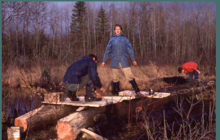
Bridge work at Red Death 1983
